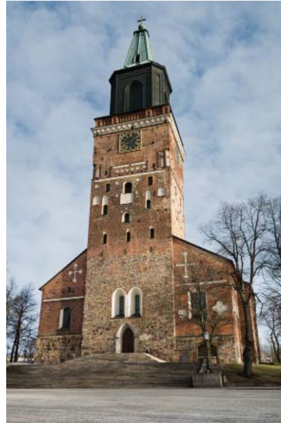
Figure 12. The cathedral is dominating the landscape of the medieval town area in the present-day Turku. The appearance of the cathedral was quite the same in the late middle ages as it is today. Photo: Lasse Andersson.
