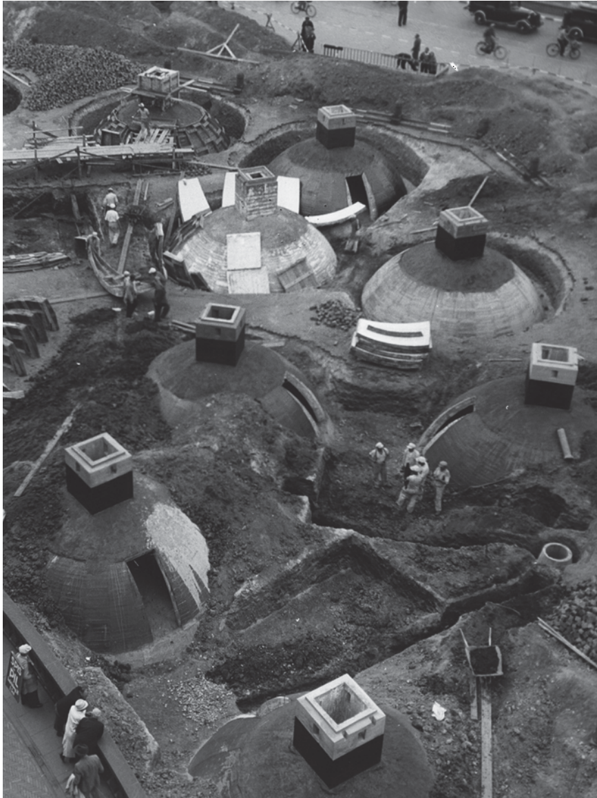
Figure 9. Photo from 1944 showing the construction work of air raid shelters somewhere at Rådhuspladsen. They explain the fragmentary patterns seen in area 2. Photo: Unknown. Copenhagen City Archive.
