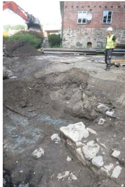
Figure 10. Parts of the wall in the 2014 trench with Hasselbackshuset in the background. The latter was built in 1814 and is one of the oldest standing houses in Uddevalla today. Mortar samples from the wall in the trench and the still standing house have been analysed in this study.
